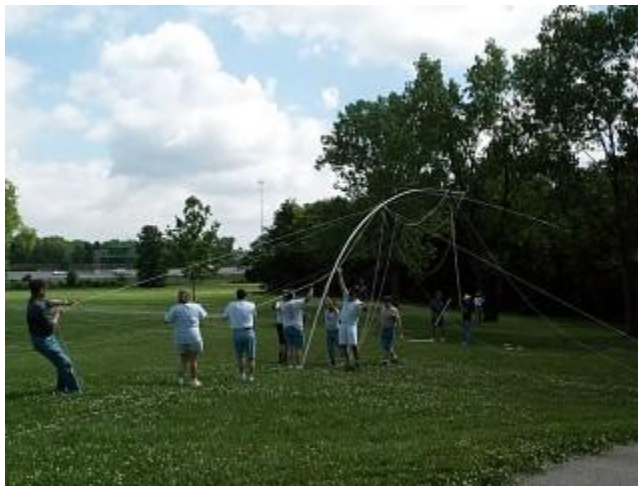
Photo 3: Continuing to raise the HF antenna, things are starting to get a little bizarre! (Note strong downward inflection of mast end.)
