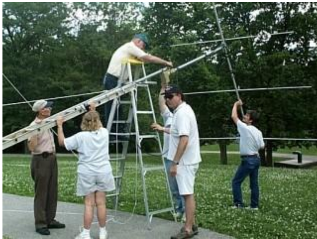
Photo 5: The team continues undaunted to set up the 6 meter beam antenna.
