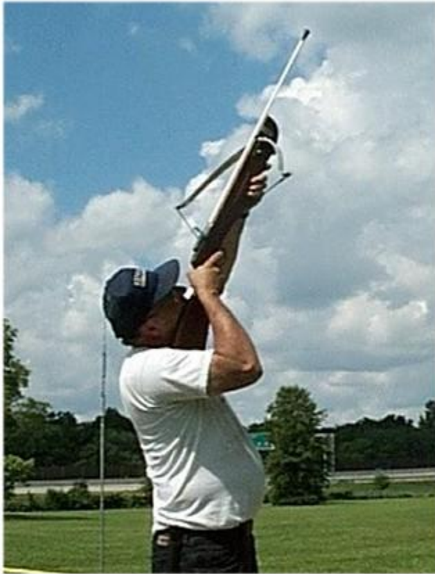
Photo 7: Don (WØDEW) takes aim with his trusty crossbow. The setup carries a monofilament fishing line over nearby treetops, allowing quick setup of wire antennas, even in 100-foot trees!
