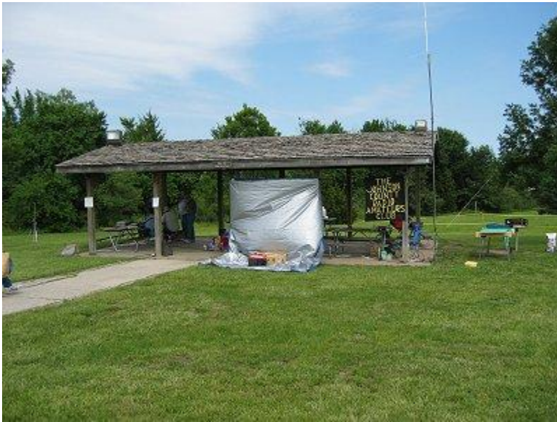
Photo 1: The Stoll park operating shelter, viewed from the west.
