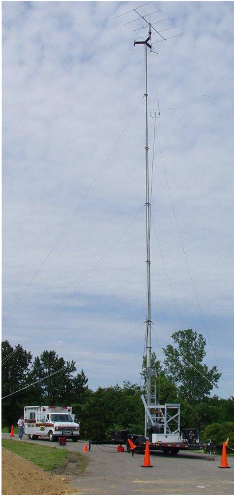
Photo 3: This photo shows the 80-foot portable tower, which carried a 6-meter beam atop and a special doublet antenna for 20, 40, and 80 meters designed by John (KOIZ). The antenna's design is unique will be featured in QST magazine in an article written by John.
